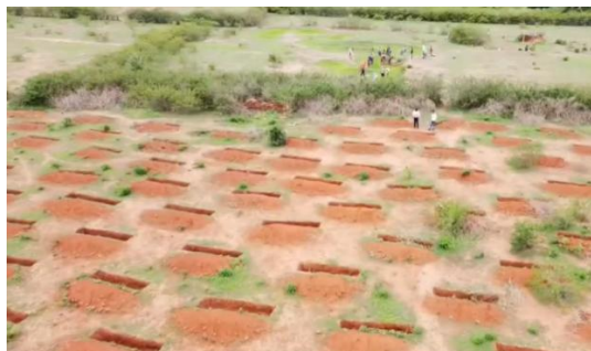
Image 6-17: Staggered Contour Trenches (SCTs)
