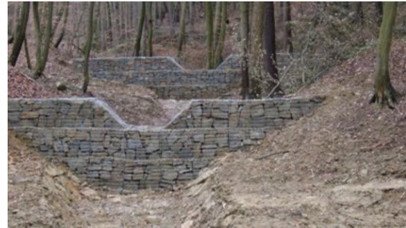
Image 6-7: Gabion Check Dam
