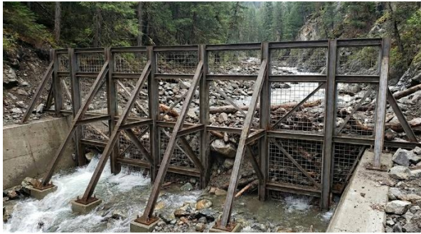
Image 6-6: Rigid steel structure
