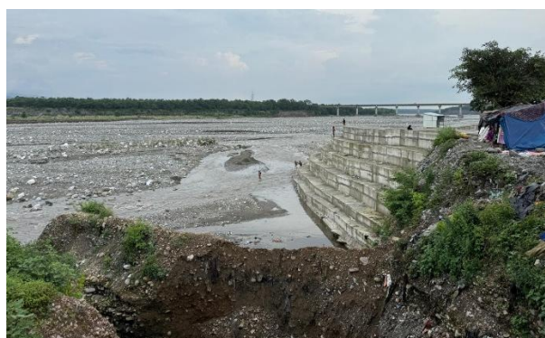
Image 6-1: Bank protection being implemented by Irrigation department at Rajpura basti
