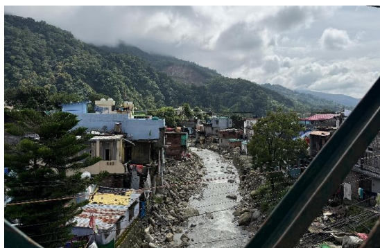
Image 6-4: Encroachment along Kalsiya Nallah
