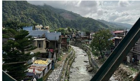
Image 6-8: Bank Protection of Kalsiya Nallah with Gabion Walls
