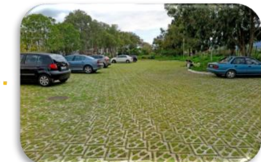
Permeable pavers in parking area
